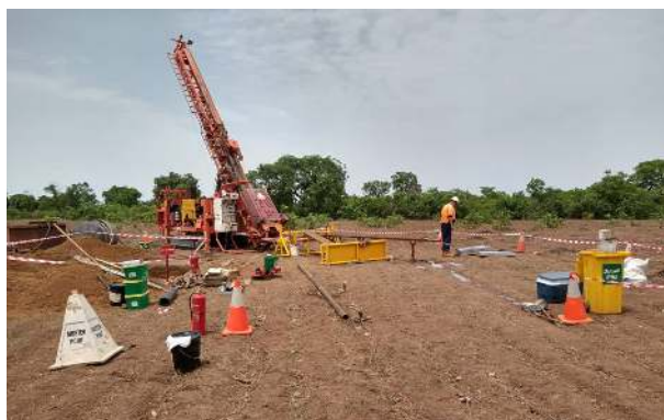
First drill pad
